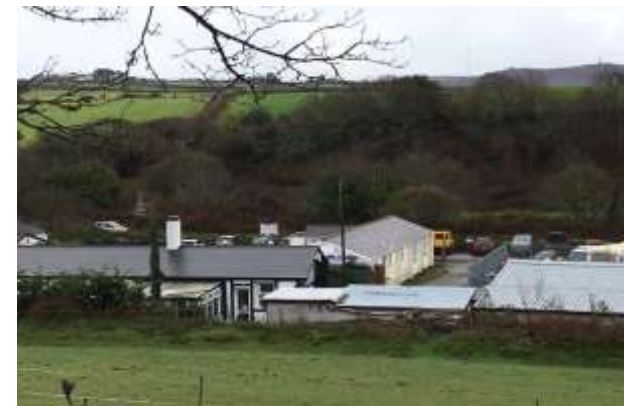
FIGURE 93 REMAINING WAAF BUILDINGS
