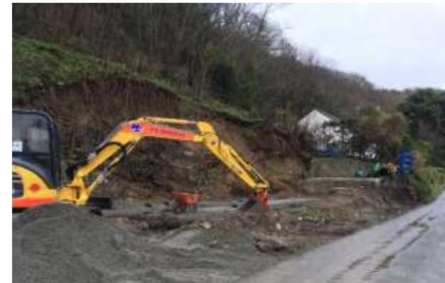
FIGURE 74 EXCAVATING PLOTS INTO THE HILLSIDE, SUNNYVALE ROAD
