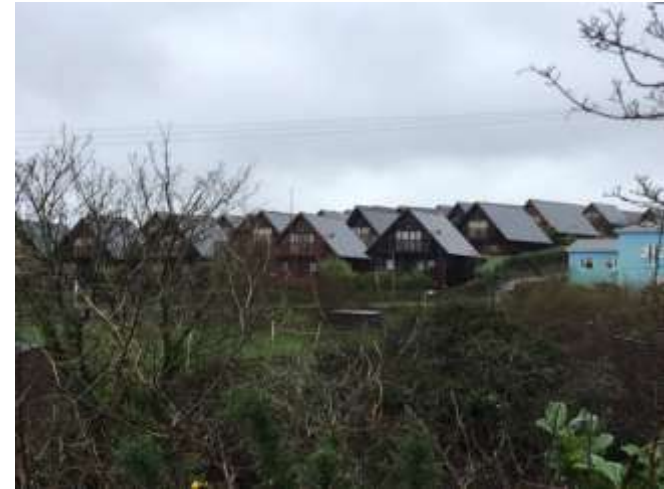
FIGURE 69 PITCHED ROOF LODGES, GWEL-AN-MOR
