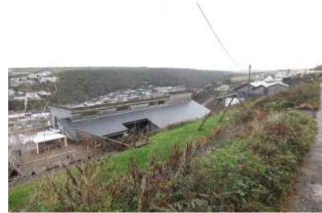
FIGURE 49 ARCHITECTURAL NEW BUILD OFF GREEN LANE
