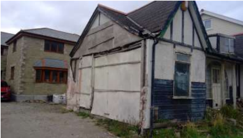
FIGURE 42 THE OLD POST OFFICE, AWAITING DEMOLITION AND REDEVELOPMENT
