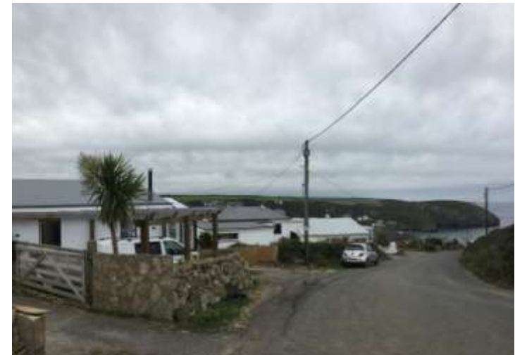
FIGURE 44 BITUMEN CLAD ROOFSCAPE OF THE 1960S BUILDINGS
