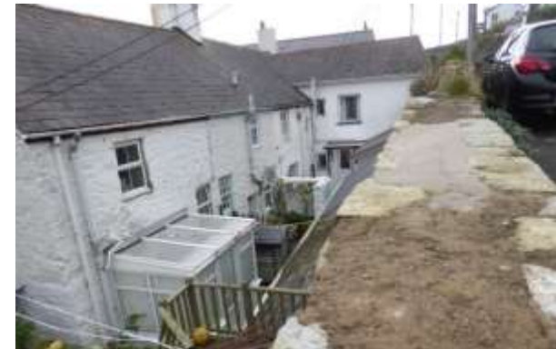
FIGURE 22 NARROW YARDS REAR OF HARBOUR TERRACE
