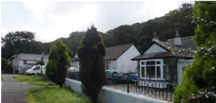
FIGURE 104 1930'S BUNGALOWS WITH BAY WINDOWS AND GABLE ENDS
