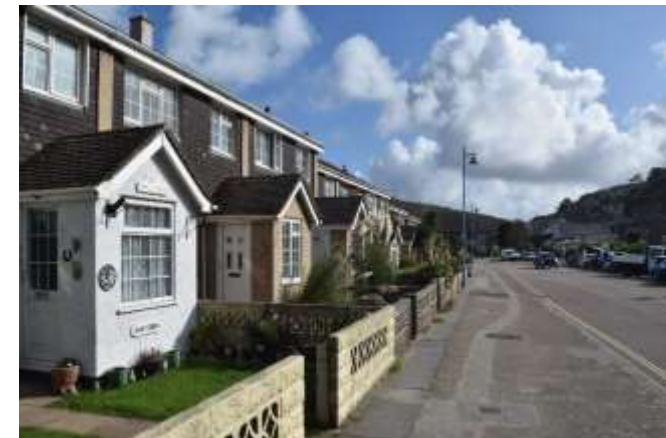
FIGURE 29 THE HARBOUR HOUSES FACING THE B3300
