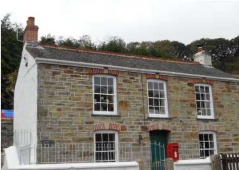
FIGURE 77 HISTORIC RIDGE TILES, LOWER NANCE
