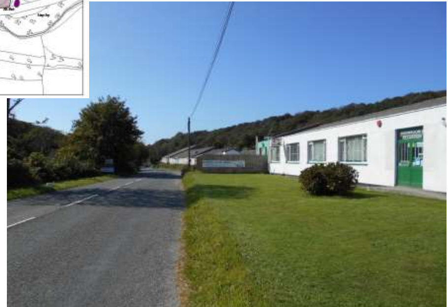
FIGURE 92 FORMER WAAF BUILDINGS ALONG THE B3300
