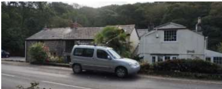
FIGURE 105 THE TIN STREAMER'S COTTAGES WITH MODERN EXTENSION
