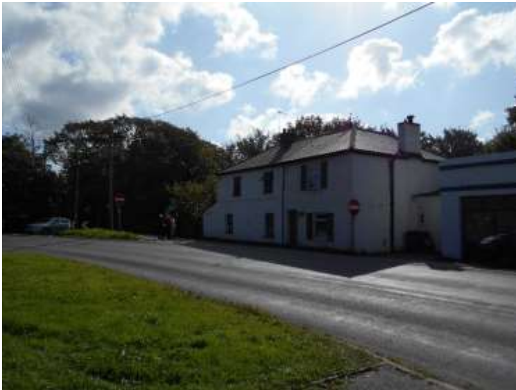
FIGURE 83 19 TH CENTURY TWO STOREY COTTAGES
