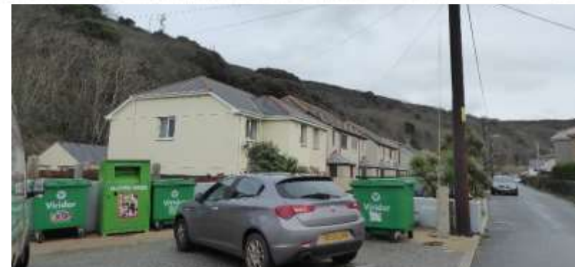
FIGURE 71 LINEAR DEVELOPMENT AT THE FOOT OF THE STEEP VALLEY SIDE
