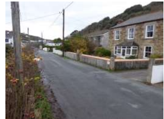
FIGURE 73 EXAMPLES OF THE DIVERSITY OF HOUSING DESIGN ON SUNNYVALE ROAD
