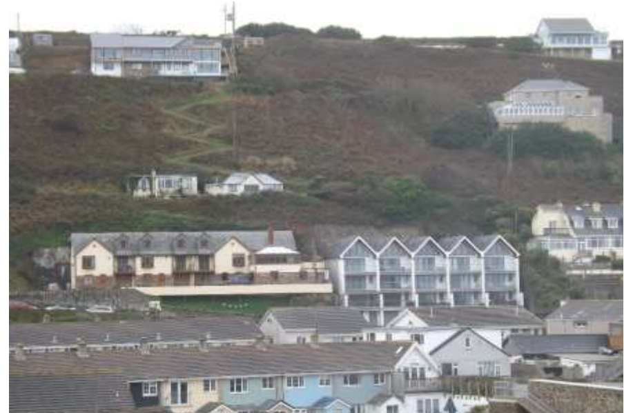
FIGURE 48 LARGE MODERN DEVELOPMENT ON THE STEEPLY SLOPING SOUTHERN VALLEY SIDE
