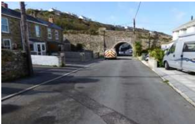
FIGURE 9 THE INCLINE BRIDGE
