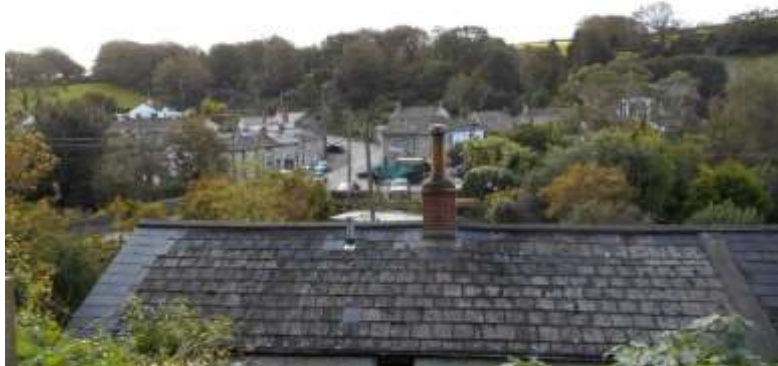
FIGURE 78 ROOFSCAPE VIEWS FROM THE MINERAL TRAMWAY
