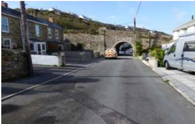
FIGURE 9 THE INCLINE BRIDGE
