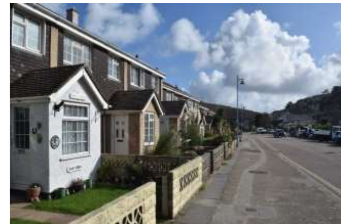
FIGURE 29 THE HARBOUR HOUSES FACING THE B3300
