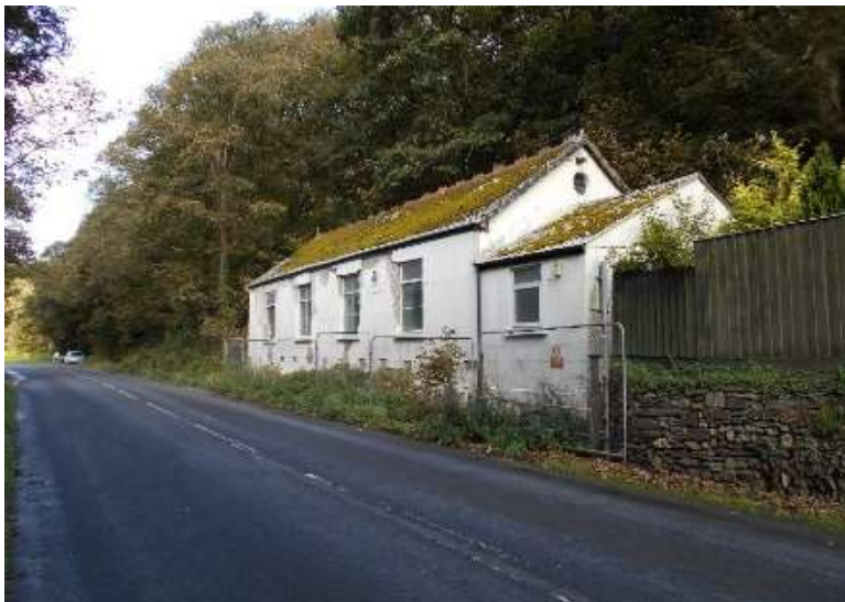
FIGURE 80 THE INSTITUTE IN DISREPAIR
