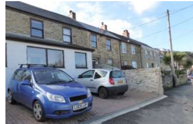
FIGURE 12 GARDEN CONVERSION TO PARKING, GLENFEADON TERRACE
