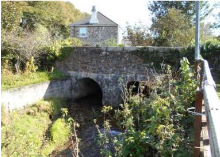
FIGURE 79 THE HISTORIC BRIDGE
