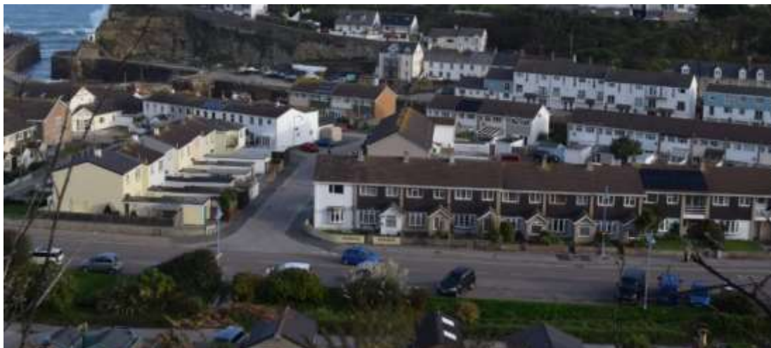
FIGURE 27 THE HARBOUR HOUSES FROM TREGEA HILL
