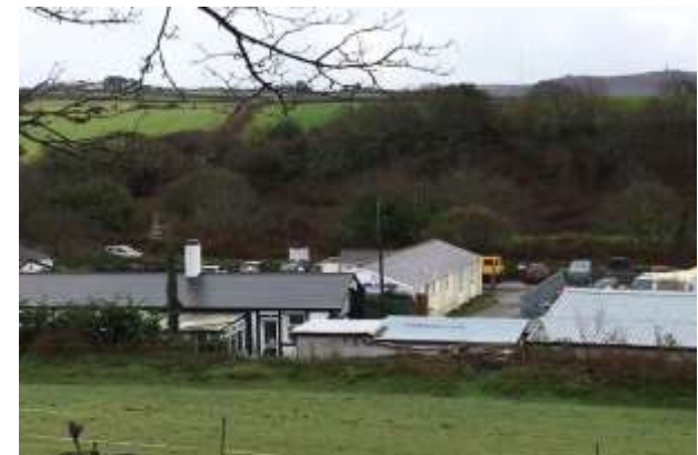
FIGURE 93 REMAINING WAAF BUILDINGS
