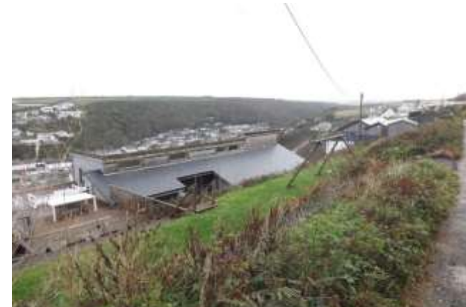
FIGURE 49 ARCHITECTURAL NEW BUILD OFF GREEN LANE
