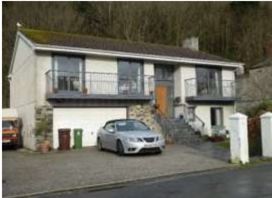
FIGURE 72 MOORFIELD, WITH STONE DETAILING
