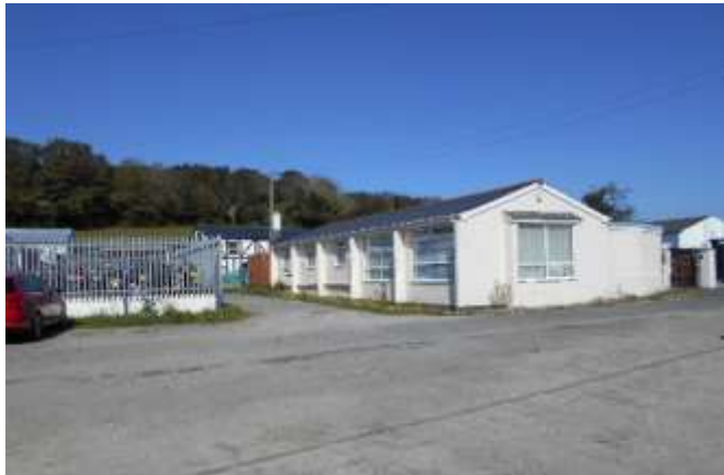
FIGURE 96 FORMER WAAF BUILDING, NOW A COMMERCIAL UNIT
