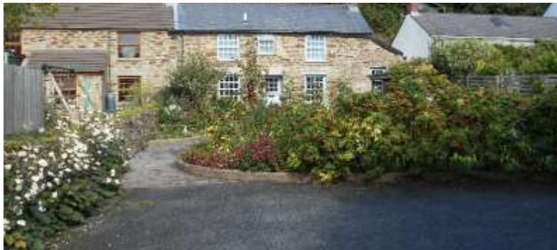
FIGURE 85 19 TH CENTURY ROW OF COTTAGES
