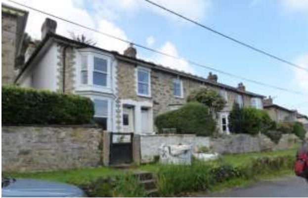
FIGURE 7 PRIMROSE TERRACE (SHOWING RAISED WALKWAY)
