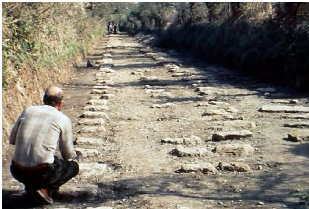
39e Surfaced tram with loop exposed..jpg
