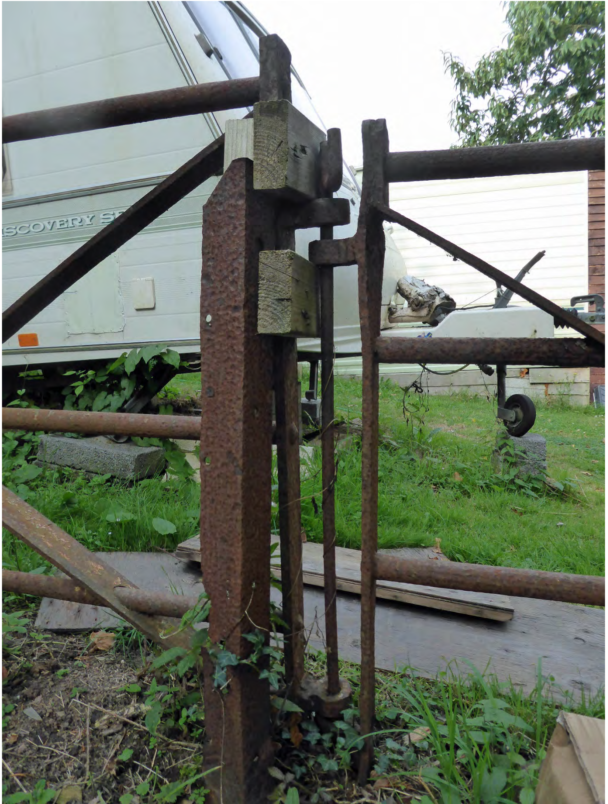
68 Iron gate hinge detail, Cambrose farmhouse.jpg
