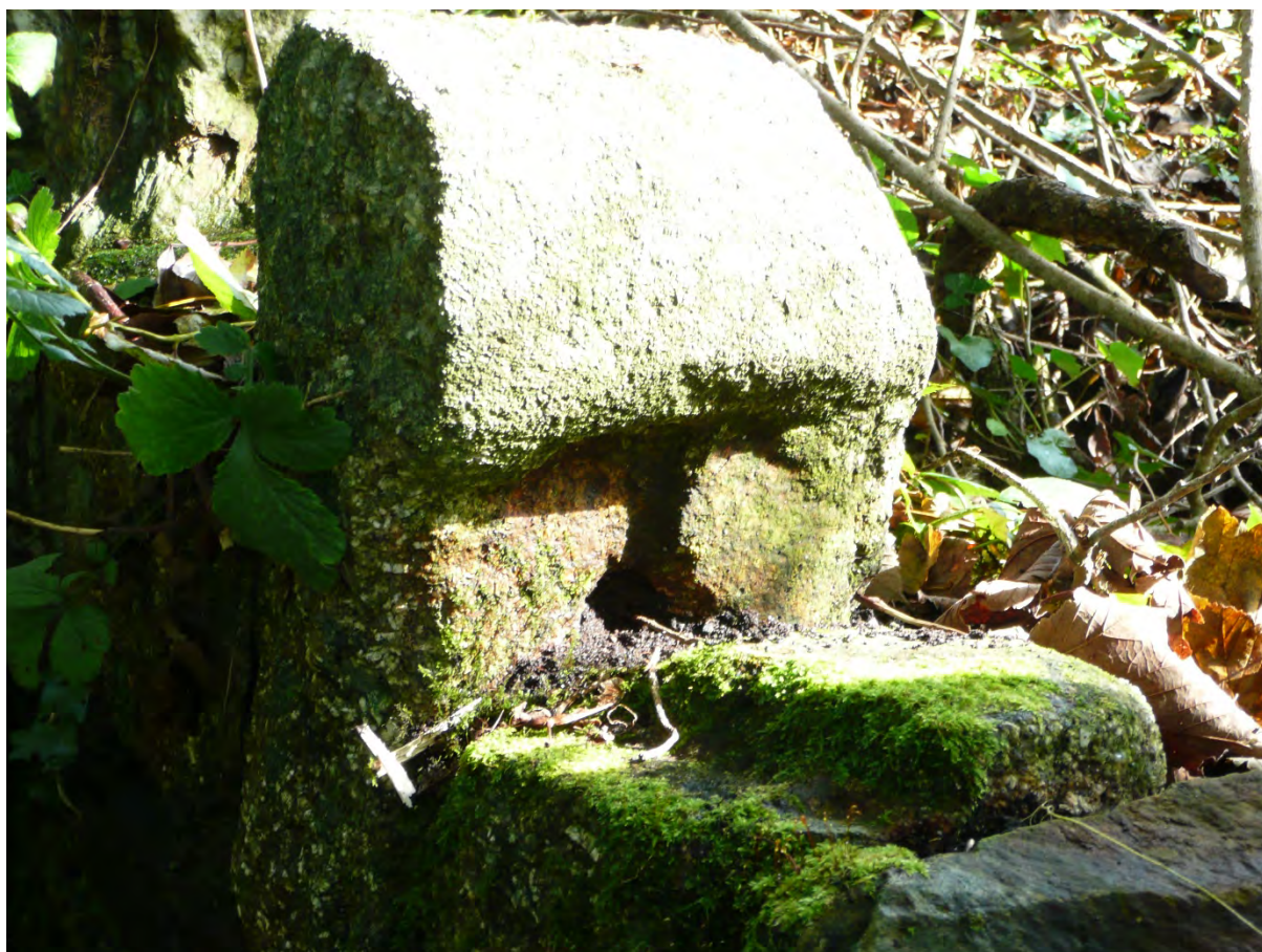
40f Sett stone in rebuilt tramroad wall.JPG
