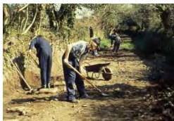
39c Exposing the setts tones by hand..jpg
