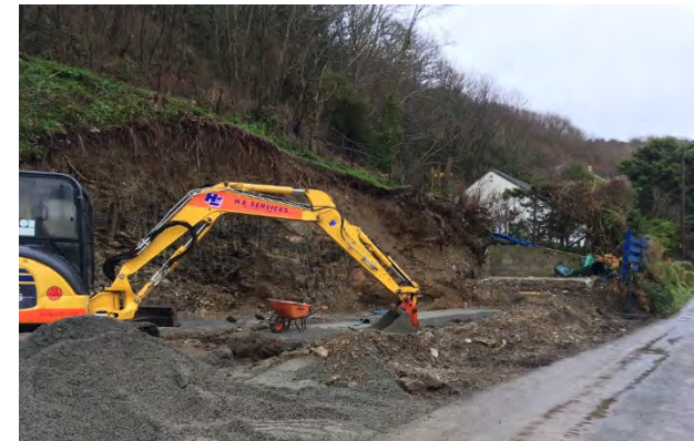
FIGURE 74 EXCAVATING PLOTS INTO THE HILLSIDE, SUNNYVALE ROAD
