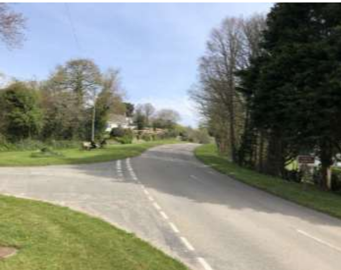
Verge at Cambrose and Conifer Stand, looking towards Porthtowan
