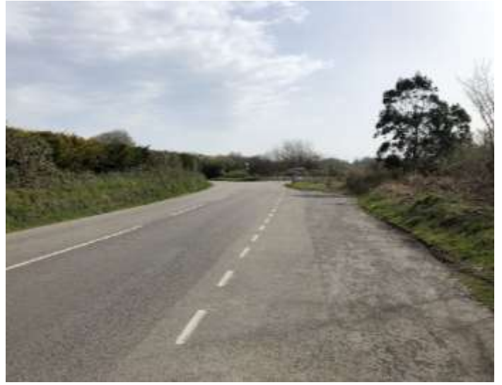
Road Bridge and Cambrose Junction with Eucalyptus
